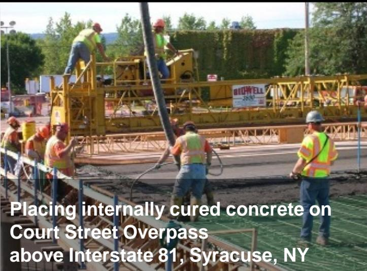
**Placing internally cured concrete on Court Street Overpass above Interstate 81, Syracuse, NY**
