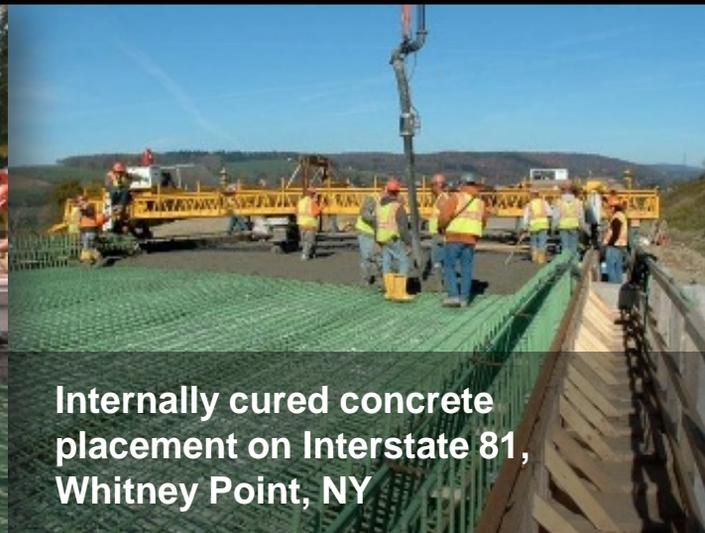
Internally cured concrete placement on Interstate 81, Whitney Point, NY
