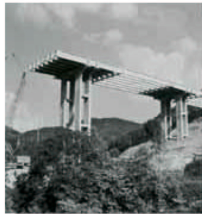
Lightweight concrete was used on the Shelby Creek Bridge to reduce superstructure weight. (Photo courtesy of PCI.)
