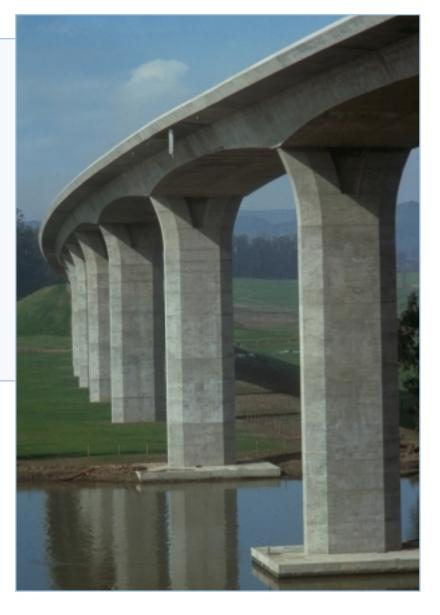
ing from 250 feet in length over the main channel, to 120 feet to the west. The bridge, which has a constant superstructure width of 68 feet, is haunched with a minimum structure depth of 7 feet 9 inches at the center of the span, to a maximum structure depth of 12 feet at the piers. The bridge piers, supported on piles, are voided 8' x 25' columns with beveled edges and soft flares at the top.
