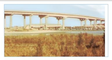
the channel opening, seemed to be the answer, except for one more problem. The US Army Corps of Engineers required that any bridge crossing the channel had to have a main span 180 feet long. This was completely unprecedented for prestressed bridge construction in Florida. Before this, the longest beam length ever used was 100 ft.
