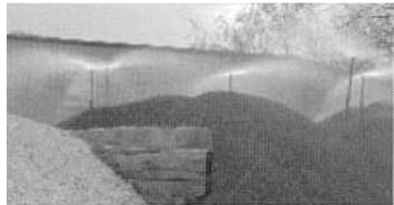
**Sprinkling Aggregate in a Stockpile**
