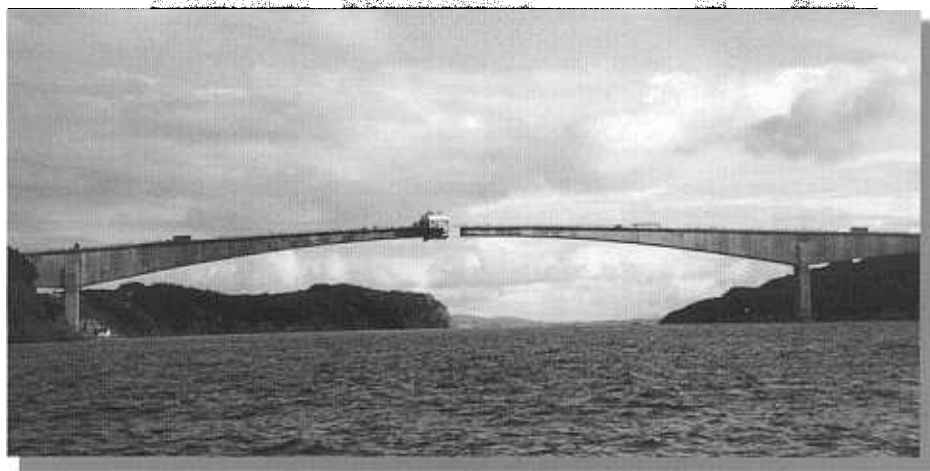
HPC lightweight aggregate concrete was used to reduce the weight of the main span on the Stolma Bridge
